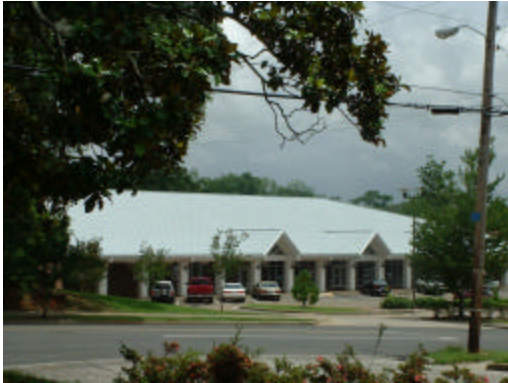
Fairhope Post Office with high albedo roof.
